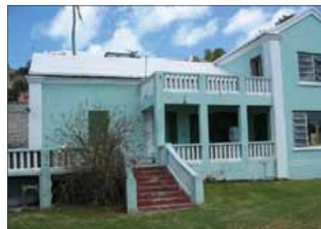
Lane School, now a Grade 3 Listed Building
