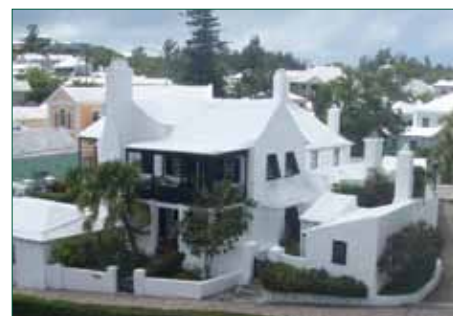
The newly painted Bridge House seen from the roof of Buckingham
