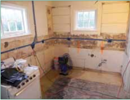
Stokes Point Mews in progress....
