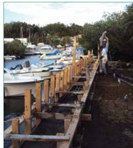
The Waterville seawall in progress
