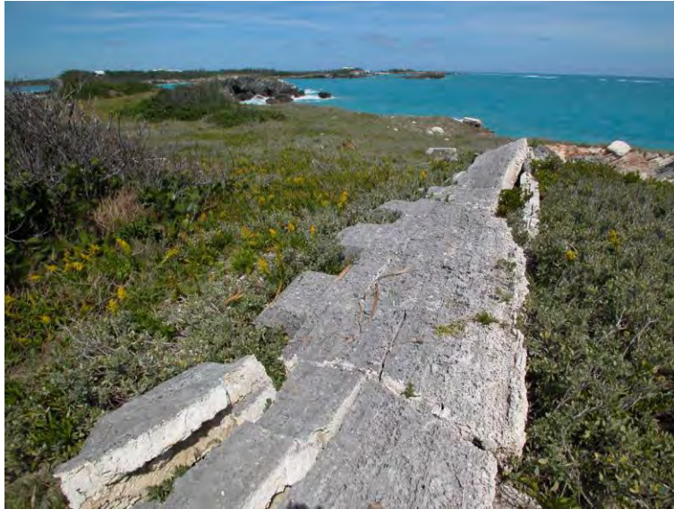
Photograph 5 showing the collapsed wall of Southampton Island Fort after Hurricane Fabian in 2003.
