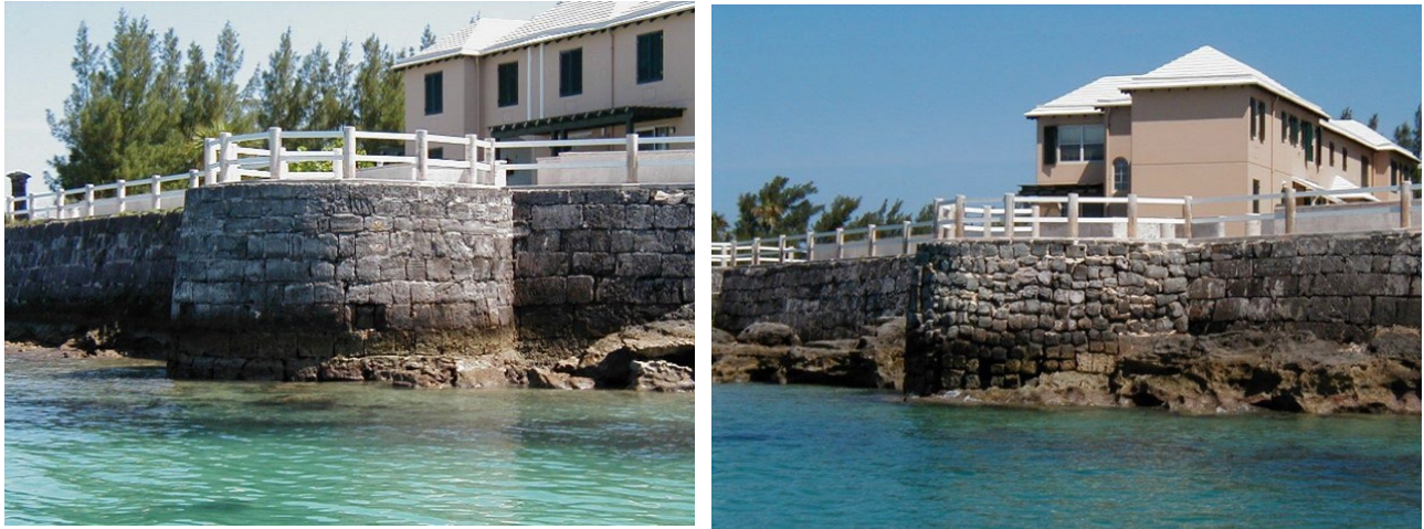
Figure 2: Bathhouses at Boaz Island look for all the world like bastions or bulwarks that are normally found at the corners of forts. Note openings that allow the sea water to enter.
