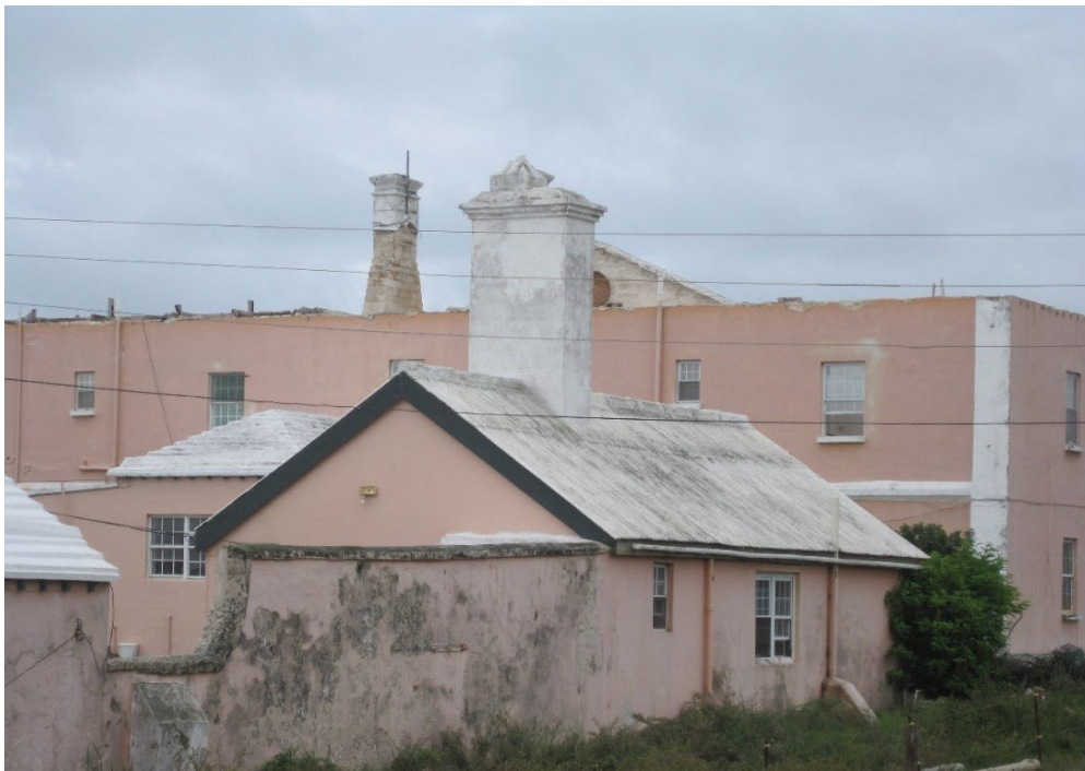
Figure 3: Seen from the rear, the building was without a roof when this photograph was taken in 2019.
