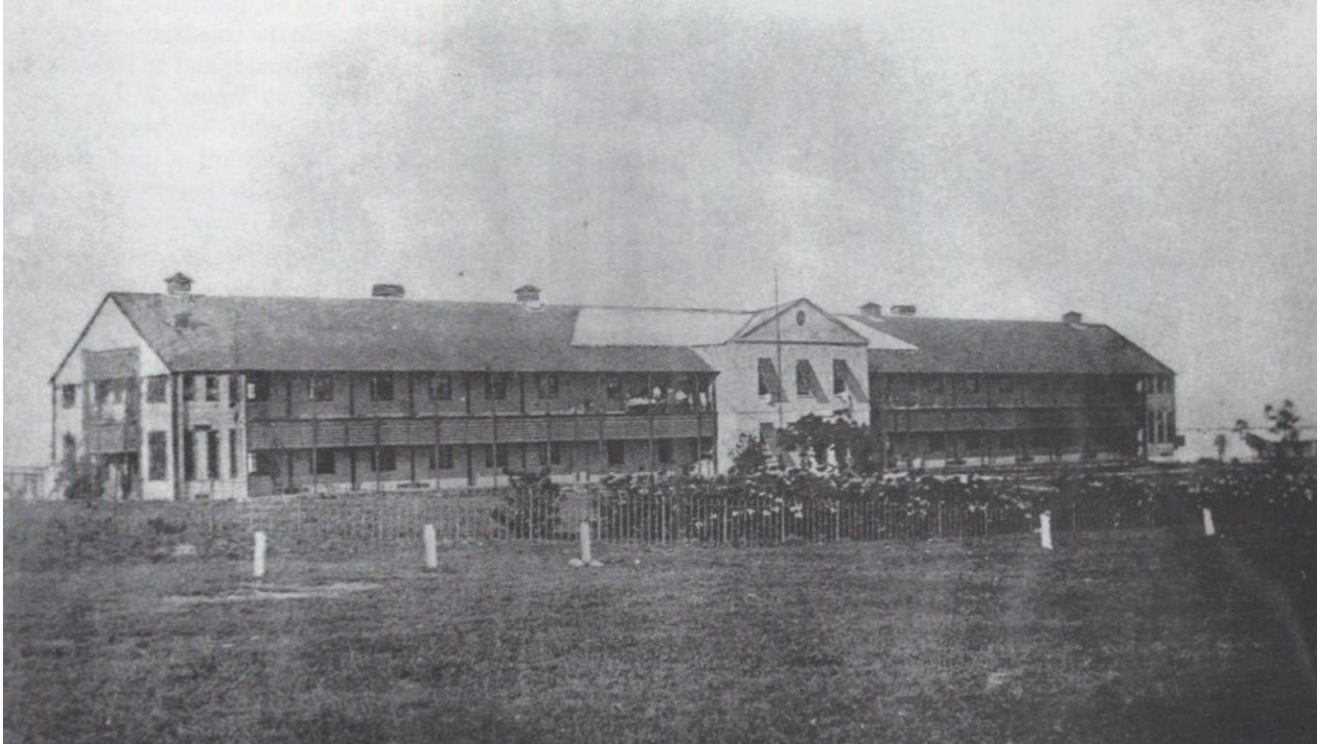
Figure 1: The earliest image is this photogravure taken around 1910 which shows the original stone Garrison Hospital with its new wooden wings and verandah. St George's Historical Society Collection, Bermuda Archives.
