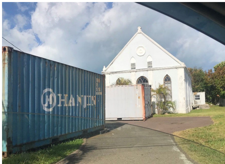
The recent addition of a third container partially blocks the view and detracts even more from the Grade 1 listed building.
