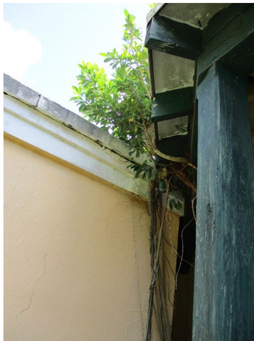
An invasive Ficus tree has rooted in the corner of the Octagon, threatening its integrity.
