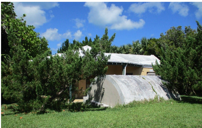
The Octagon and its large domed water tank in 2022.
