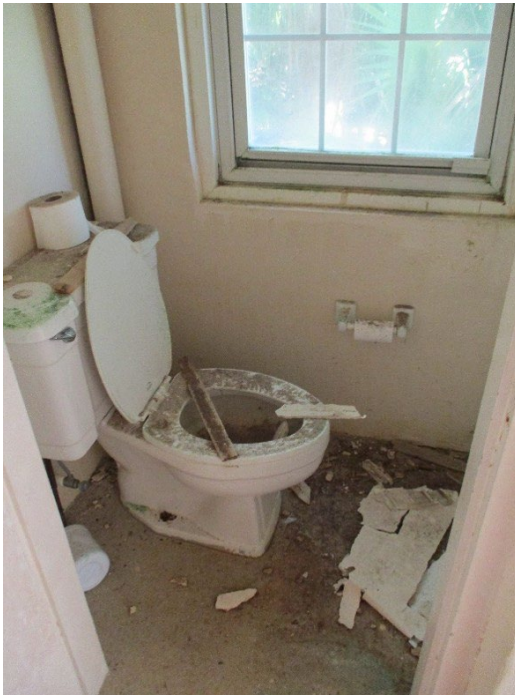
There are presently no working toilets on the island for tour groups. The visitor's restroom is unusable as the ceiling has caved in, the water tank that serves it has been cracked by tree roots and the pump is broken.
