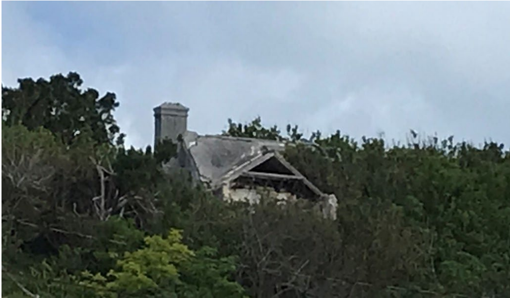
The Ratteray Homestead today is totally dilapidated and beyond saving.
