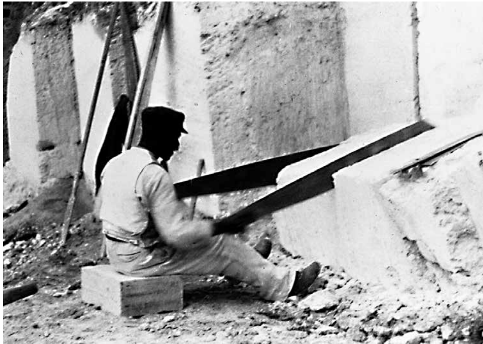
A skilled stonecutter masters his tools cutting large limestone blocks. The chisel in the background would have been used to create primary channels in the rock face.
