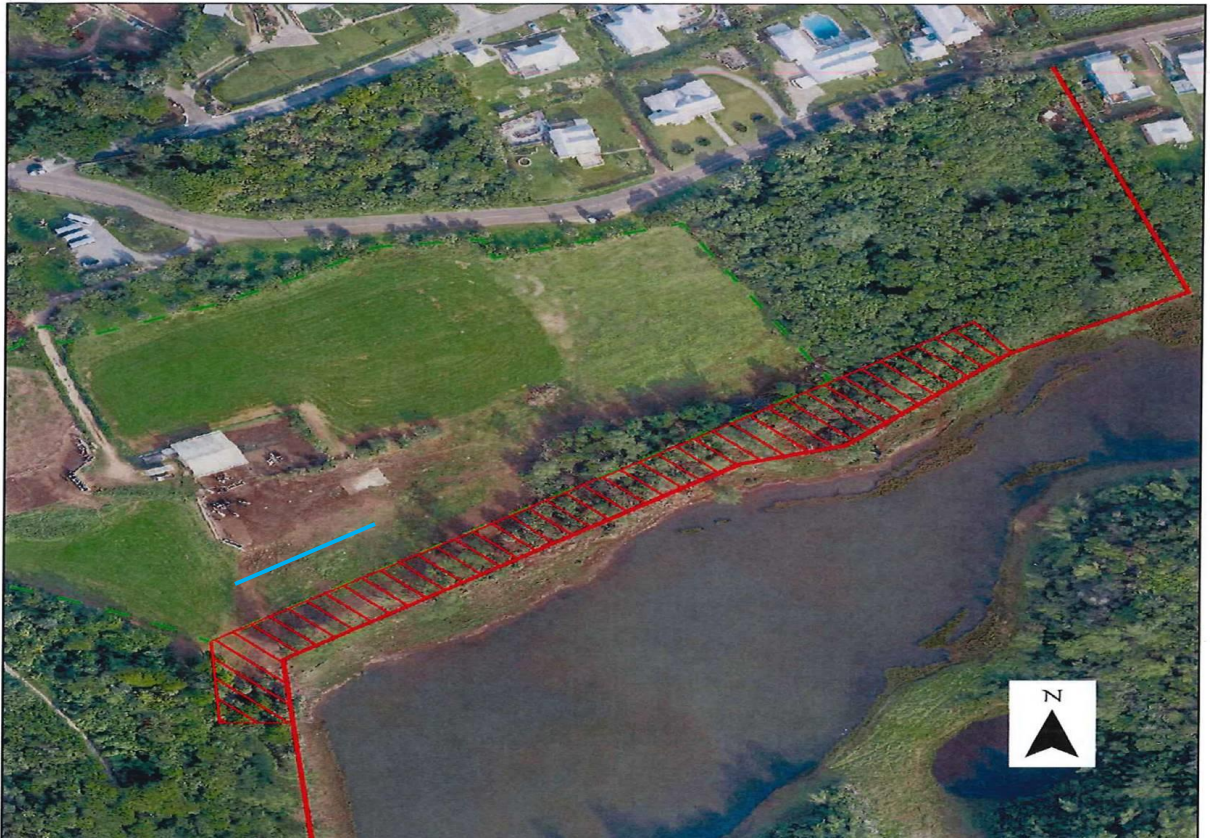
Figure 17 Shows the area of land owned by government that is designated as nature reserve that will be included in the proposed work. Repair of fencing, some invasive removal and all the berm and ditch marked in blue will be developed on this section of land owned by the government of Bermuda. A letter has been provided by the appropriate minister and the department of the Environment and Natural Resources.
