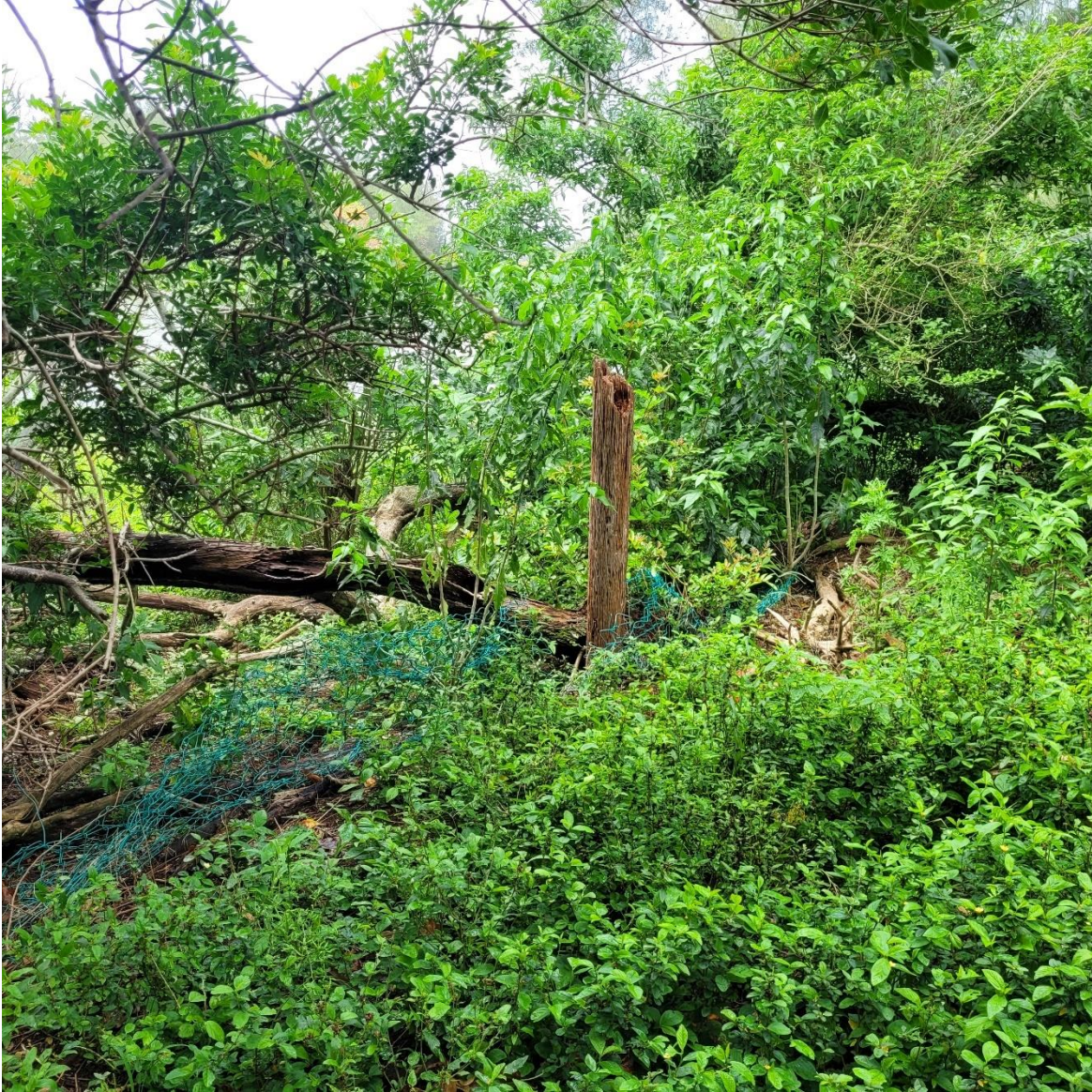
Figure 6 Damage to existing fence from trees impacted by recent hurricane activity.
