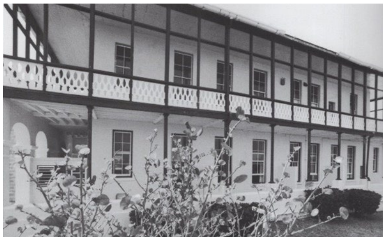
An otherwise plain building, Lefroy House's outstanding feature is the verandah on three sides of it. The east verandah is supported by metal columns. Photograph taken in 1999.
