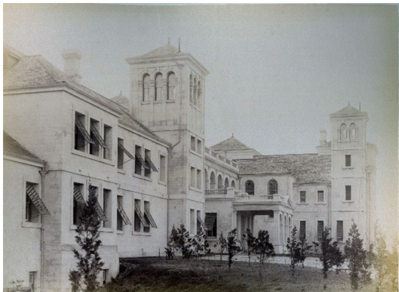
Government House had been completed by the time this photograph was taken by visitor Colonel John A M Passmore in 1899. Courtesy of the Bermuda Archives.
