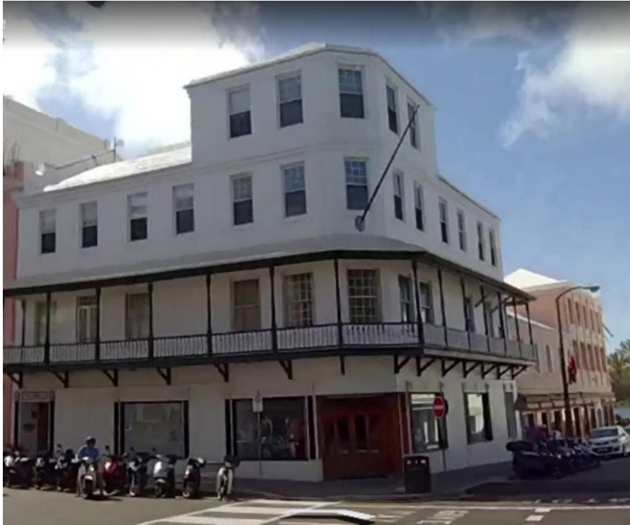
The building is already enveloped in scaffolding in anticipation of the removal of the balcony so this photo is courtesy of Google Earth.
