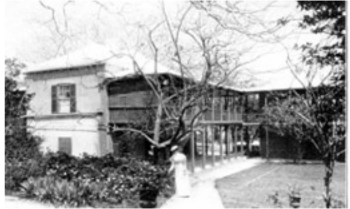
The balconies of the two buildings are connected by a bridge on the upper floor. An outside staircase was removed in 1958. Murray Jordan Album (circa 1890s), Bermuda Archives.
