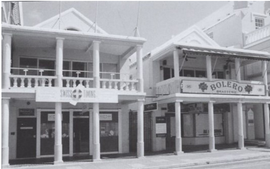
The wooden verandahs had long been replaced by concrete but Henry Hunt's two warehouses were still structurally the same when photographed about 2014.
